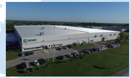
Kentucky Logistics Center (U.S.A.)
