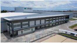
M-SENKO Logistics Center (Thailand)
