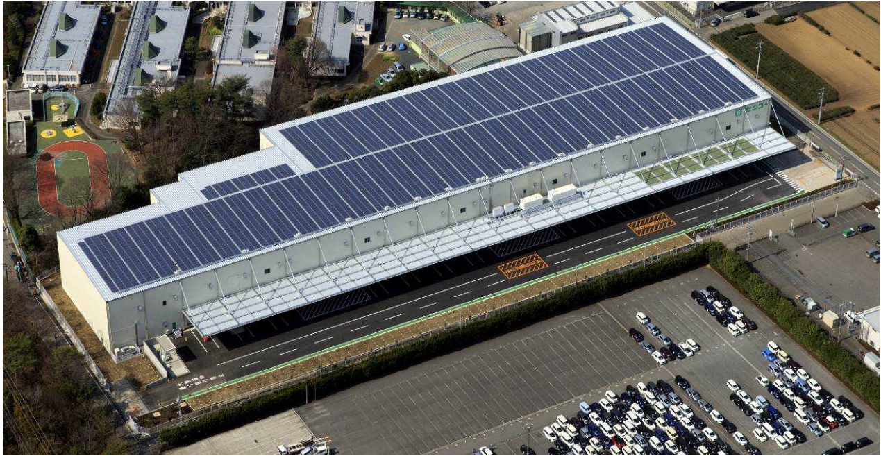
(Solar panels on the roof)
